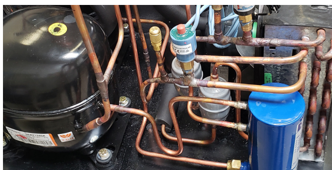
Mechanical refrigeration construction
