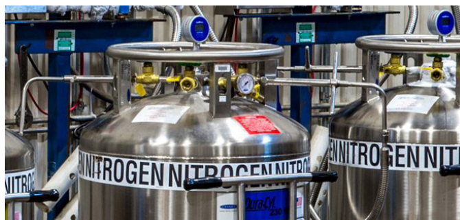
Cryogenic dewar for liquid nitrogen
